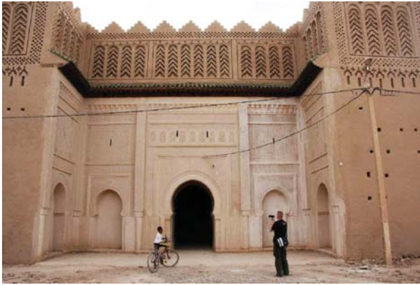
Image 6. The main entrance of the ksar of Ouled Abdelhalim
