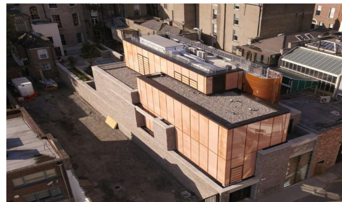
Goethe Institut Dublin / Henschion Reuter Architects (2014)
