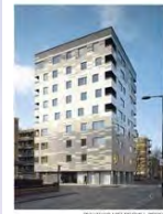
THE BUILDING BLOCKS The panels, made of three or five layers, are up to 6 inches thick and 30 feet long. But thicker and bigger panels can be made.
