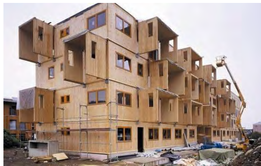
THE BUILDING BLOCKS The panels, made of three or five layers, are up to 6 inches thick and 30 feet long. But thicker and bigger panels can be made.
